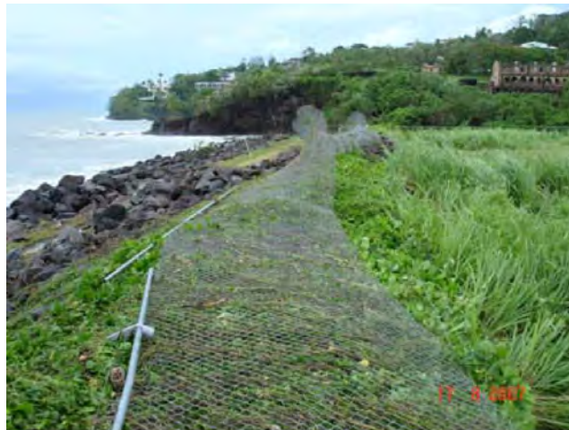
Figure 5-2 Damage to Fence at George F.L. Charles Airport
