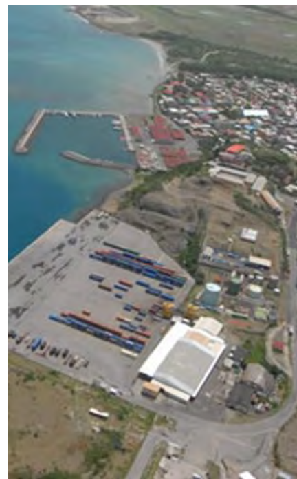
Figure 4-14 Port Vieux Fort (Source: http://www.slmtl.com/ )
