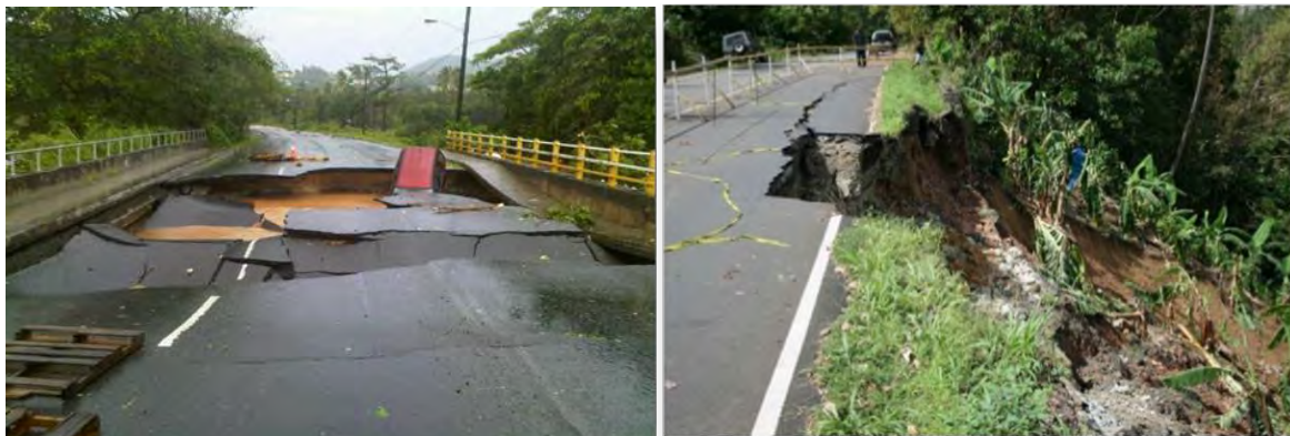
Figure 5-4 Left: Damage to the Choc Bridge caused by Hurricane Tomas – the bridge connects the north of the island to Castries (Source: Kimberly Mathurin - https://internationalmedicalcorps.org ); Right: Landslide in Barre D'Isle showing compromised north-south (Source: APESL, 2010)
