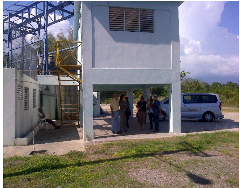
After a major flood, a pumping station in Santo Domingo was raised by the height of a person to avoid future impacts. (Source: ICF)
